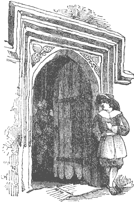
Belfry Porch, Elstow.
